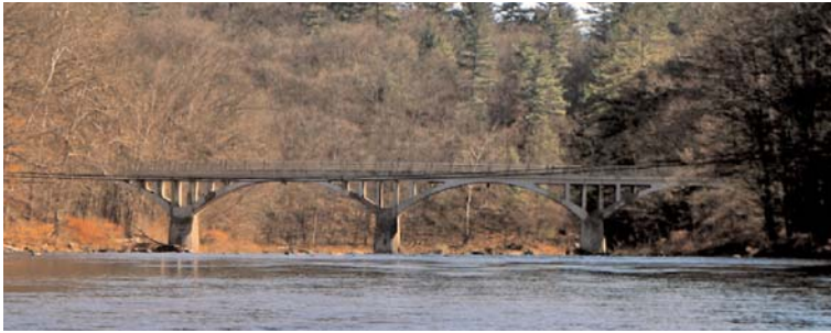
Remembering an Esopus icon, Five Arches Bridge, which is no more. Photo by Ed Ostapczuk.
