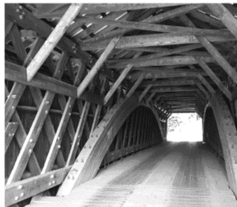
Sullivan County Park of the Month: Livingston Manor Covered Bridge Park
