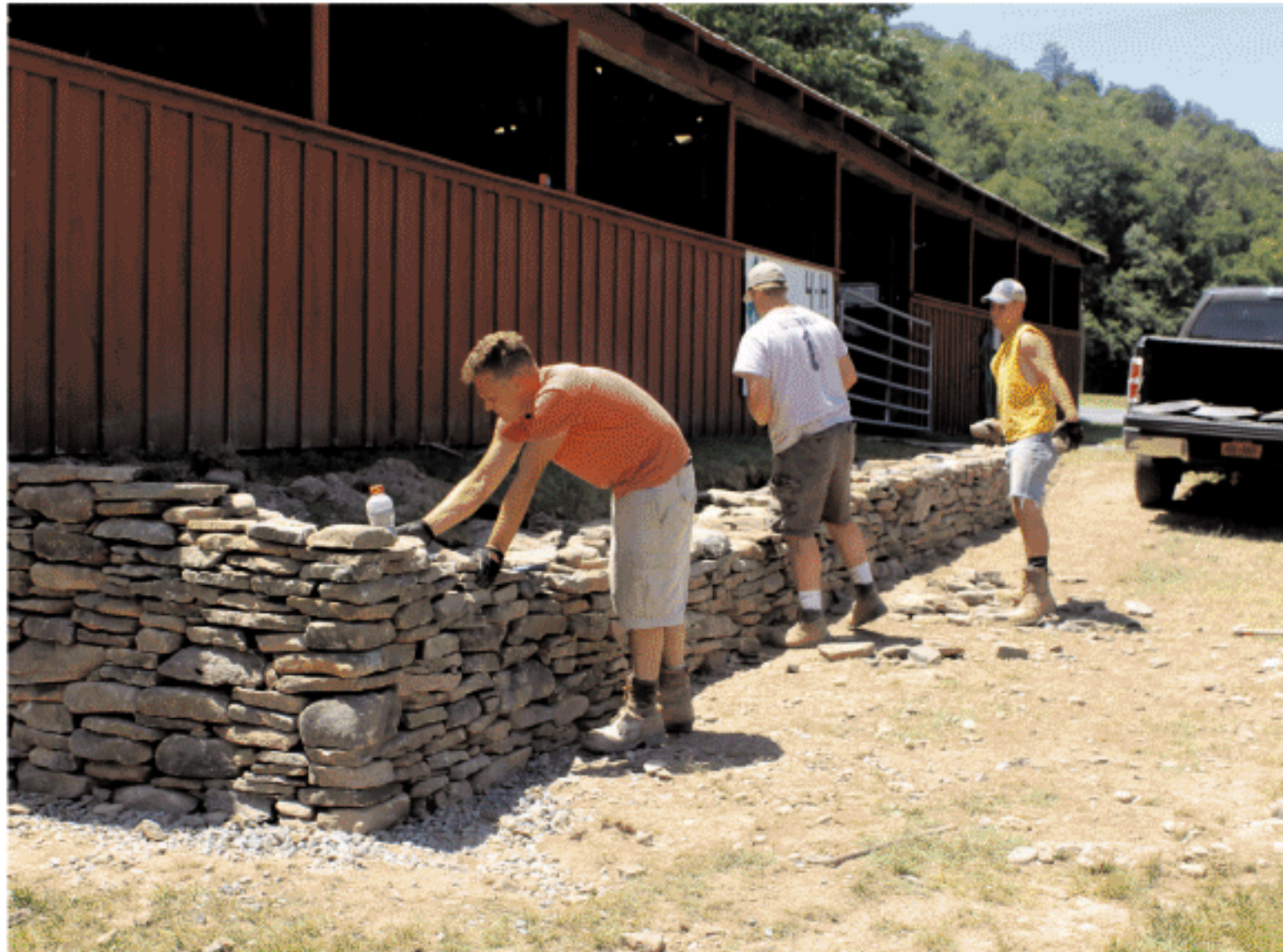
Crew from Darder Stone Works Lay Wall
