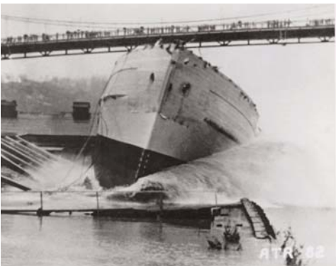
"The hull for rescue tug ATR-82 slips sideways down the ways on Rondout Creek producing a large wave as onlookers view the launch from high in the background on the Wurts Street Bridge."
